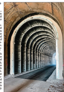
Galvanized steel was installed in the Greer Tunnel by Swank Construction to reinforce the concrete passage as part of the Montour Trail Council's three-phase renovation project. Swank will extend the ceiling-liner to the western portal beginning in spring 2024.
